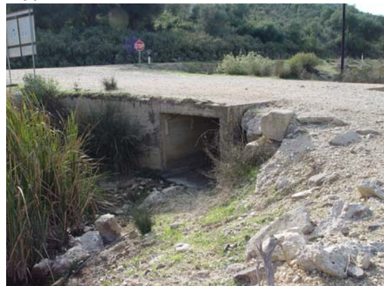
Fig. 6. Culvert under road connecting the ditch (site 55, left) with the Springs (site 56).
