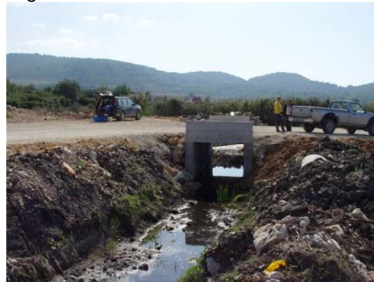
Fig. 4. The point of convergence of the drainage canal with the Glyfa springs.
