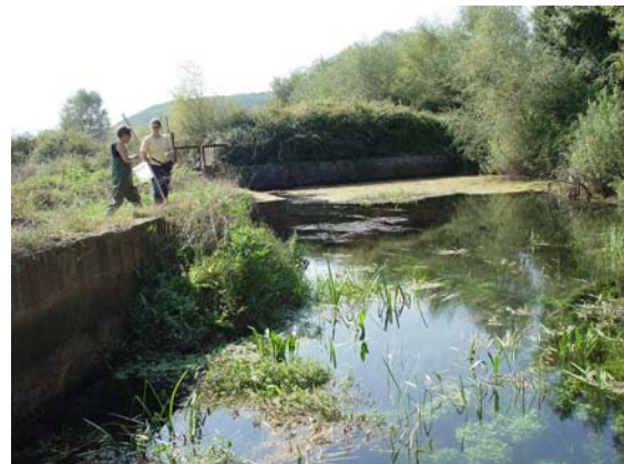
Fig. 10. Site 61 with water cress-like plants and fallen dead reeds (top).
