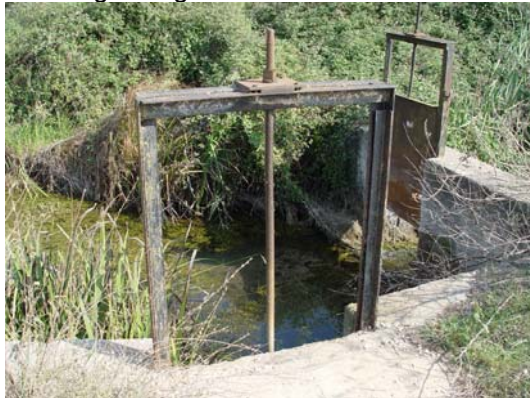
Fig. 3. The flow of the water is regulated by a system of sluices.
