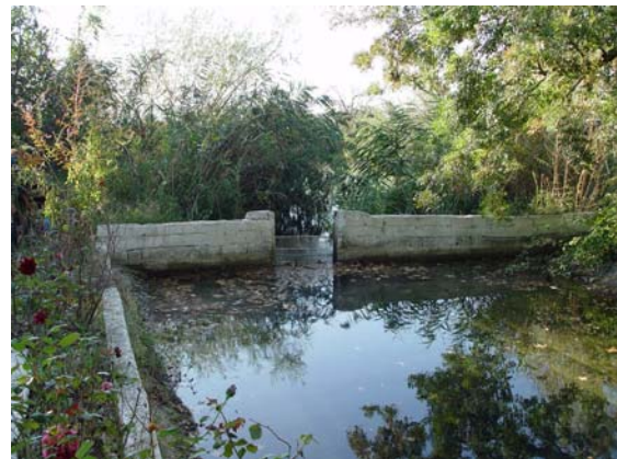
Fig. 14. Pond (site 63) and gate to prevent the trout dispersal in the stream.
