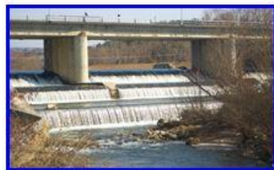
Irrigation dam Toxotes
