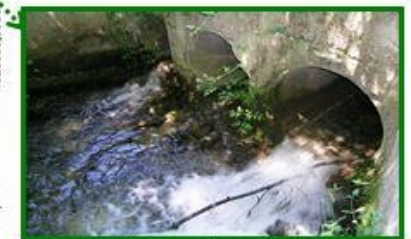
Culvert Miloy Rema
