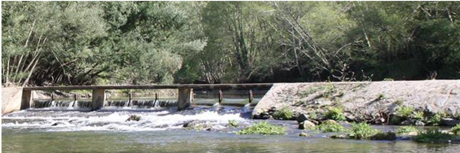
low slope weir water passes over with no waterfall
