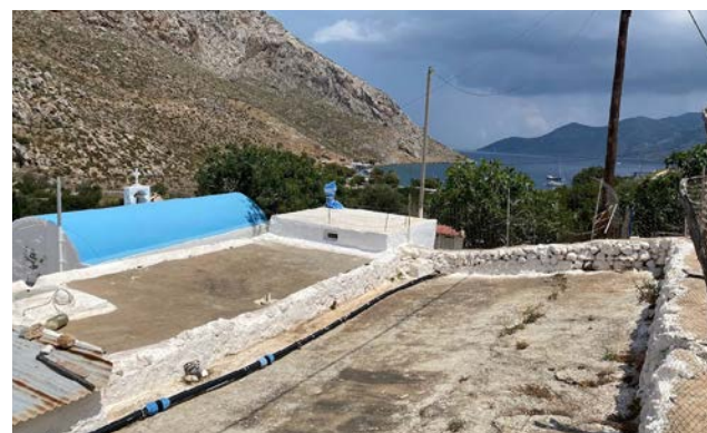
FIGURE 31 Sloping roof in Kalymnos for rainwater collection (Photo: Eugenia Tsianou).
